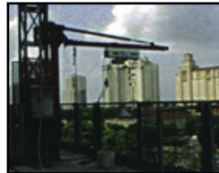
Left: Beta Max Gemini Plus Hoist on Hek Mast Climbing Work Platform.
