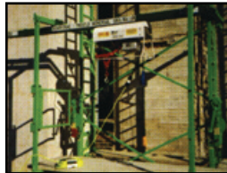
Right: Beta Max Gemini Plus Hoist on Non-Stop continuous climbing scaffold.
